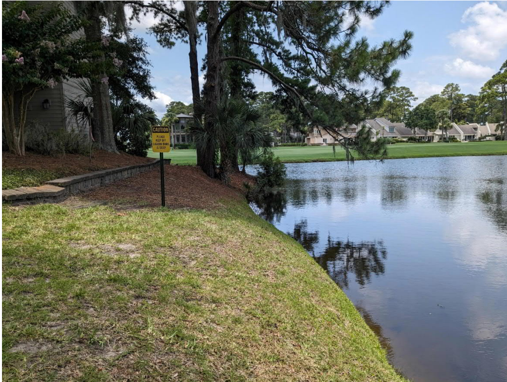
Photo 3: Slope beside Villas 186-190
