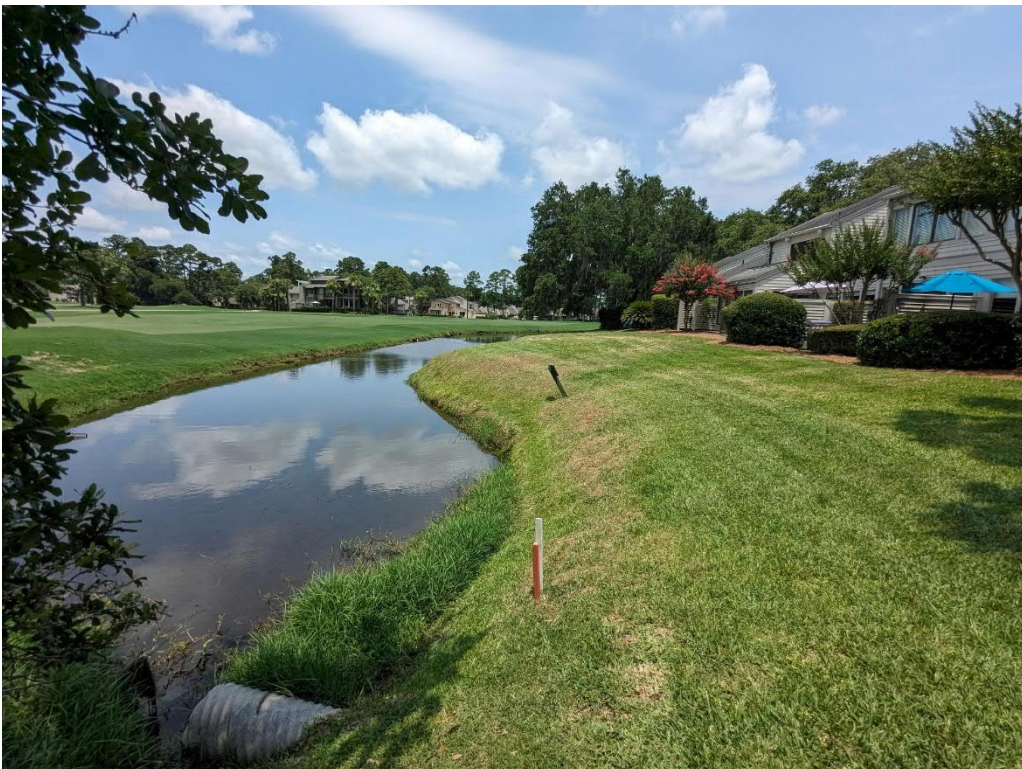
Photo 2: Slope behind Villas 181-185
