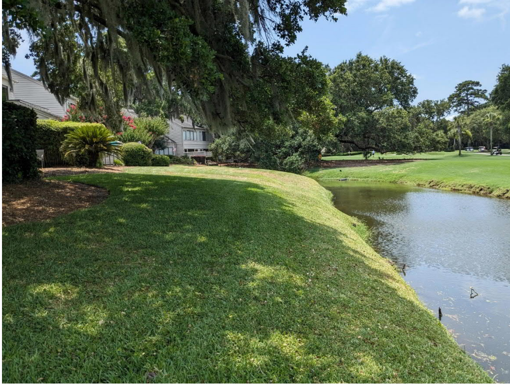
Photo 1: Slope behind Villas 181-185
