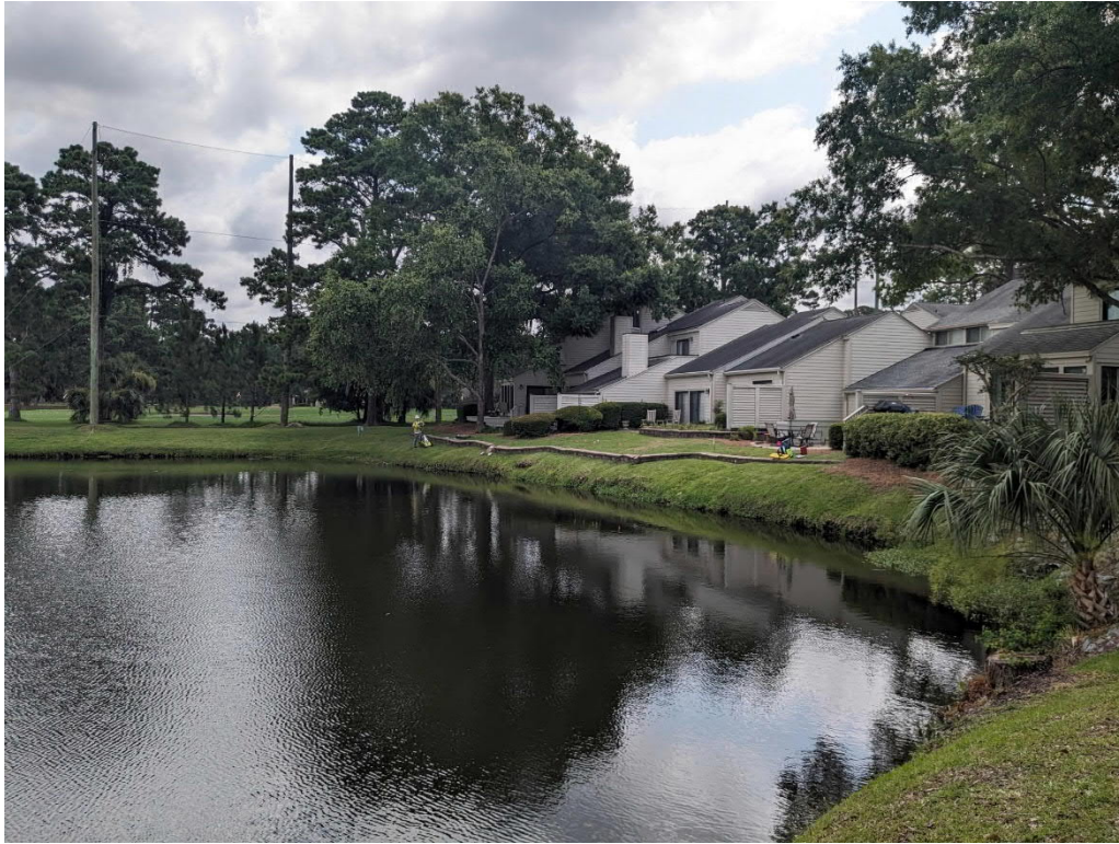
Photo 5: Slope behind Villas 191-195
